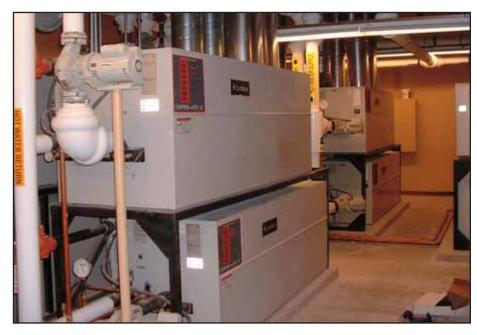
The ventilation systems were designed to operate with 100 percent outside air to ensure proper air quality. With an outdoor design temperature of 29Þ F in the winter, this application required a fairly large boiler plant.
